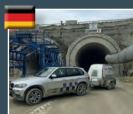
stuttgart railway line stuttgart 21
